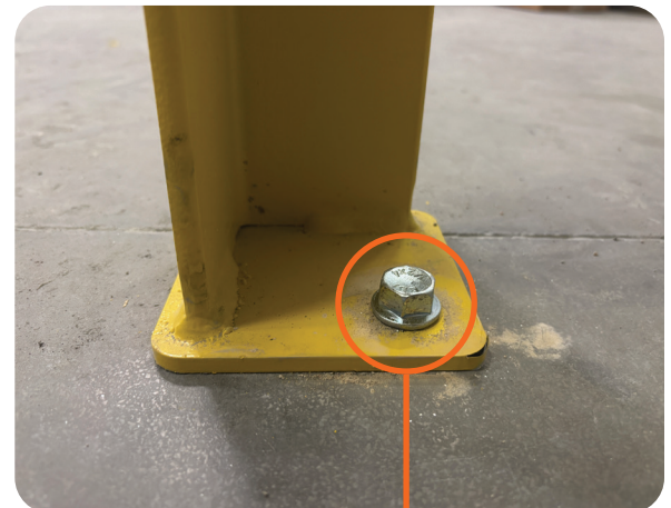
Anchor Bolts Flush with Stair
